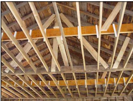
The ceiling rafters and joists have been strengthened and straightened.
