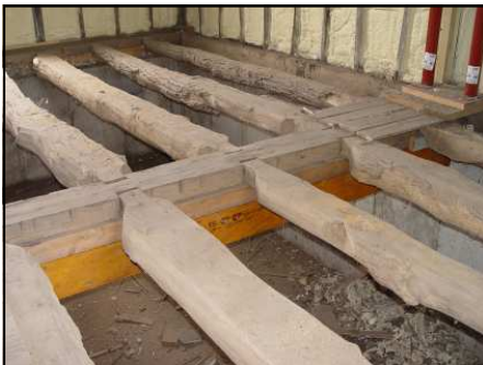
Construction methods have changed since 1852.
