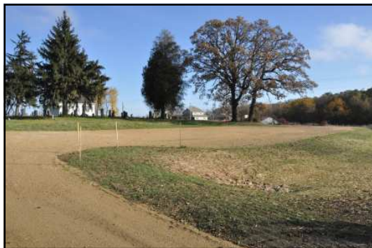
The driveway and parking lot are now leveled and graveled.
